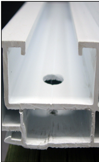
1. Pre-drill window frame.
